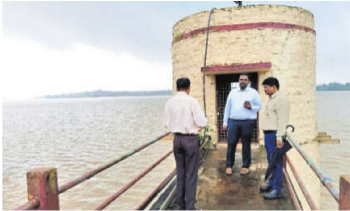
BCC Commissioner Karthik M. inspects the Rakkaskoppa Reservoir
